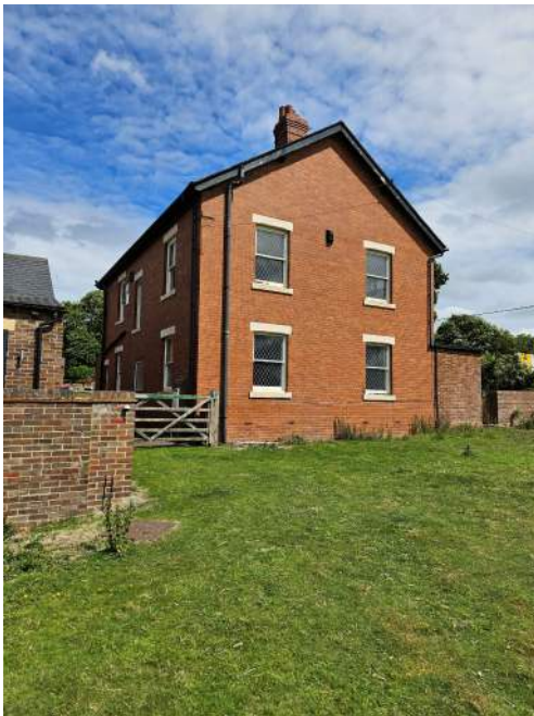
Fig 2 existing gable elevation facing field
