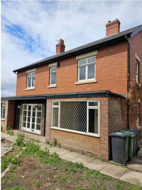
Fig 1 existing front extension with flat roof and casement windows
