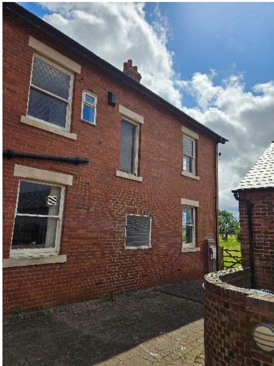
Fig 4 existing rear elevation and proximity to neighbouring property and public access
