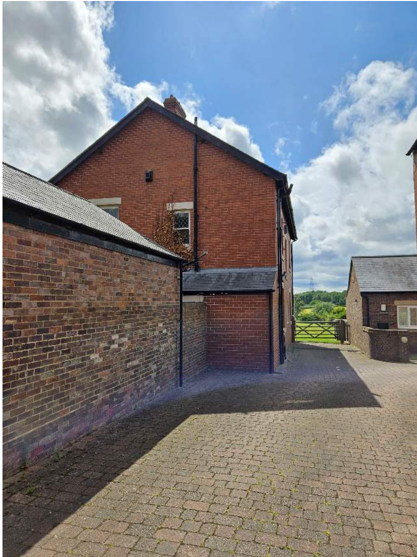
Fig 5 view down rear of the building which is tight on boundary to access to neighbouring properties.
